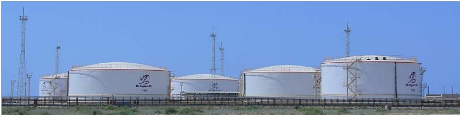
Above: Storage tankers.
